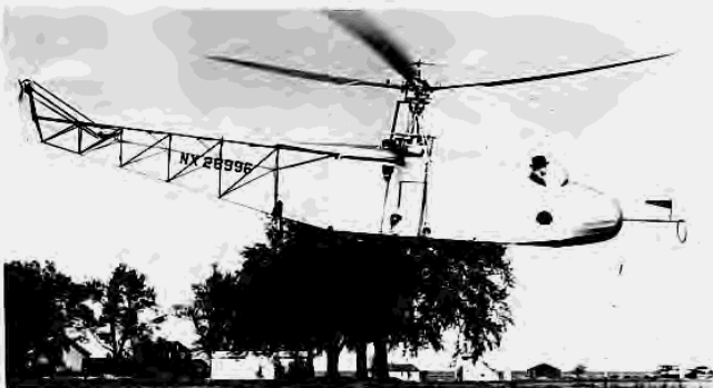
Fig. 1-3. The Sikorsky VS-300 established the modern helicopter, single main rotor configuration in December 1941 (photo from author's collection).
