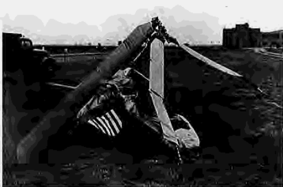
Fig. 2-11. The Kellett XR-2 autogyro before and after ground resonance in 1941 [7].
