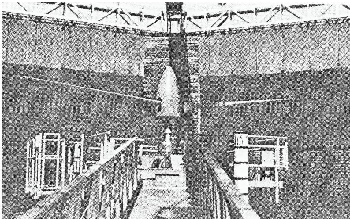
**Figure 6.** XV-15 metal-bladed proprotor tested in hover on WADC Rig #3.
