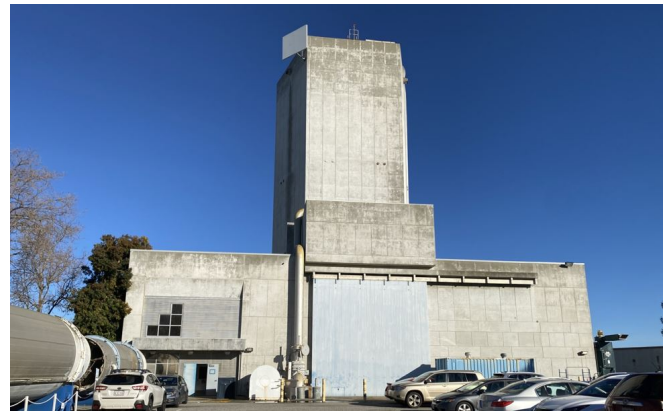
Figure 6. PAL; low pressure test chamber is contained within the tall rectangular tower.
