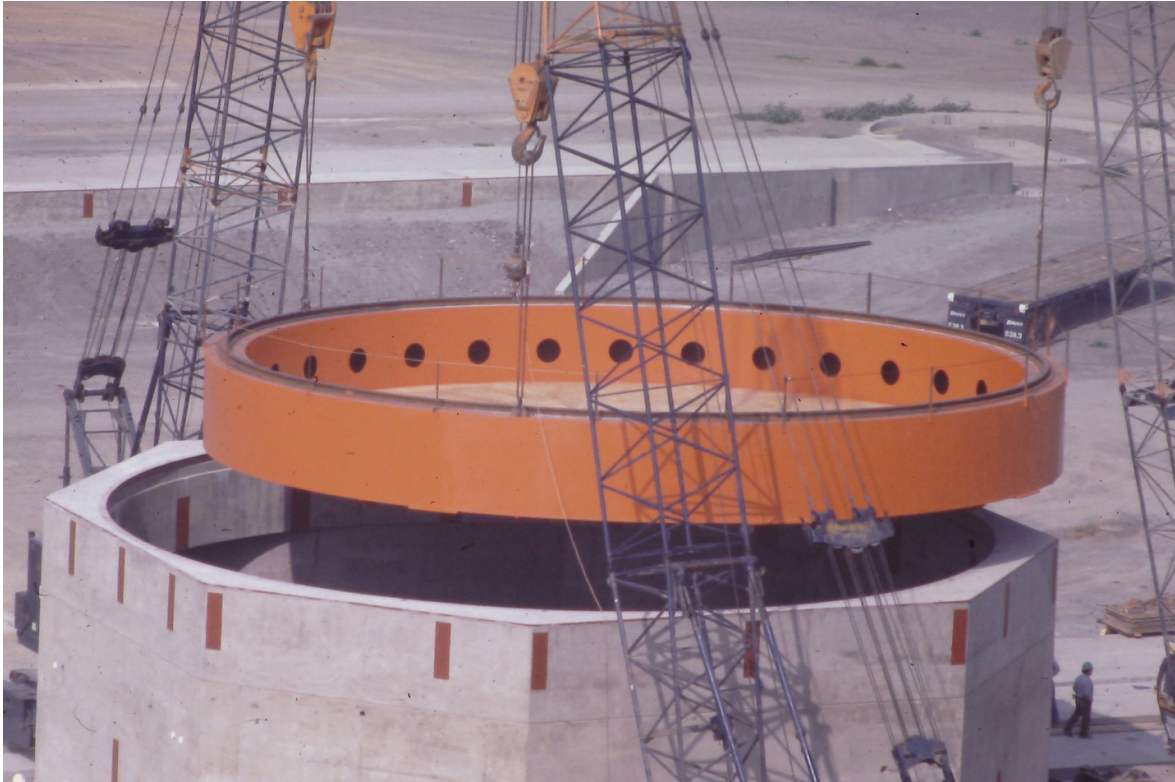
Figure 34. Lowering the turntable into the octagonal foundation. (Author's collection, KM38)
