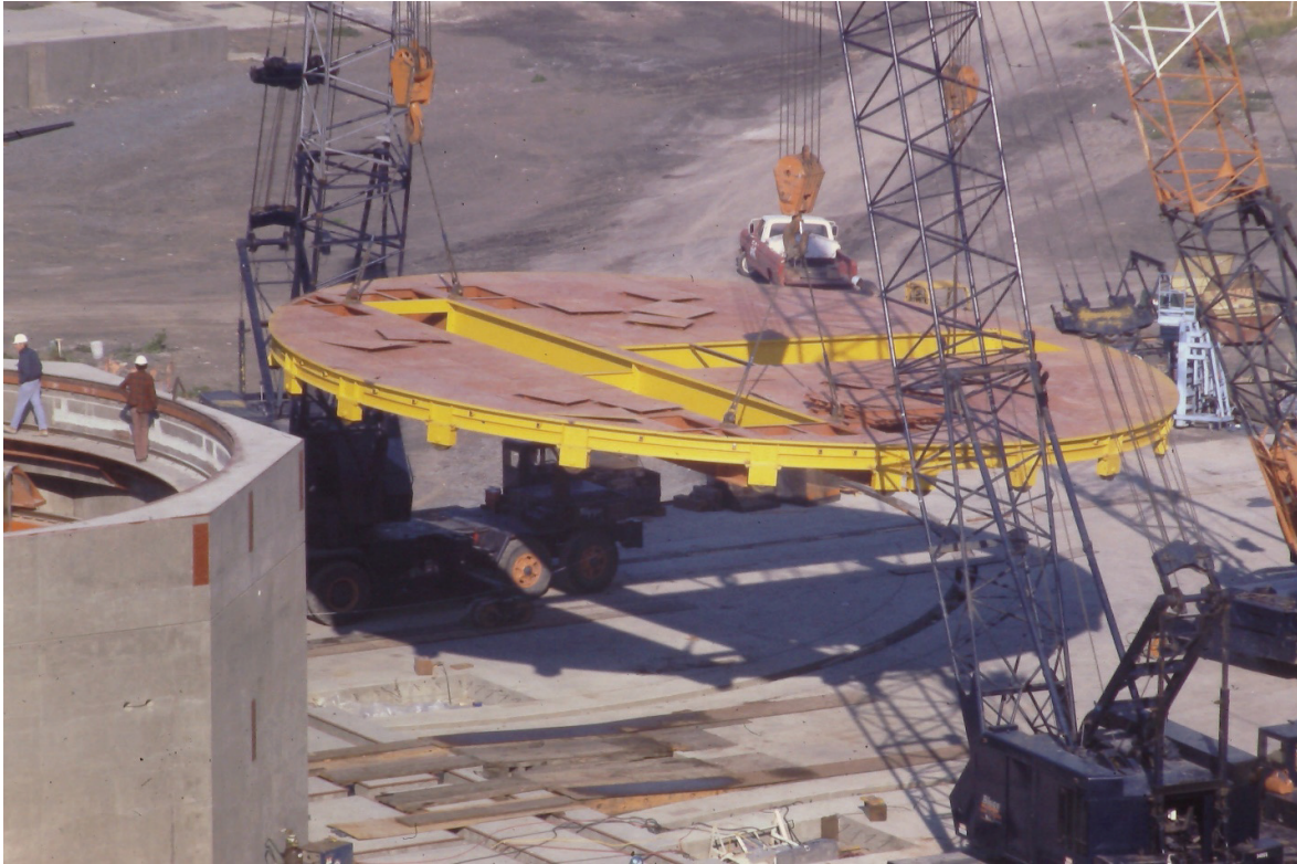
Figure 36. Lifting the turntable floor for installation. ( T.J. Forsyth collection, TJ3 )
