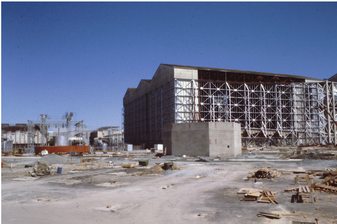
Figure 33. Completed octagonal concrete foundation for the model support and balance. ( Author's collection, KM34 )
