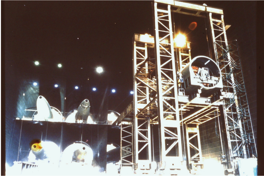
Figure 50. Last drive unit partially lifted with the elevator. ( Author's collection, KM25 )
