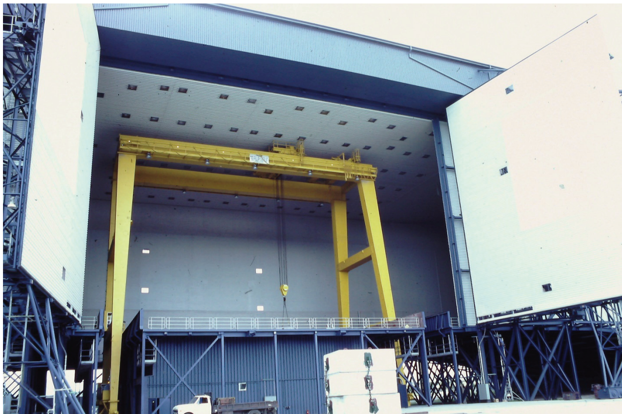
Figure 44. Model-handling gantry crane in the 80- by 120-foot test section with the test-section doors and floor access panels open. (Author's collection, KM76)
