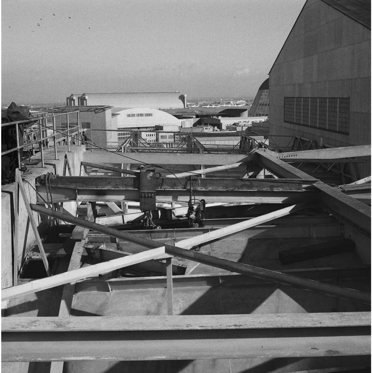
Figure 24. Top of drive that was to be repaired with hatch cut, and installation of a portable trolley and crane to enable fan removal. (NASA A71-8826)
