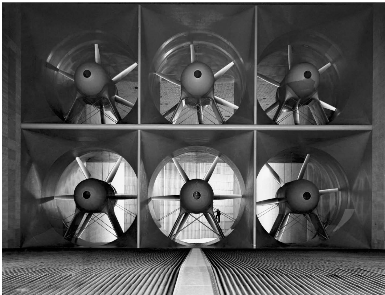
Figure 20. Completed six-fan drive. ( NACA AAL-5993 )
