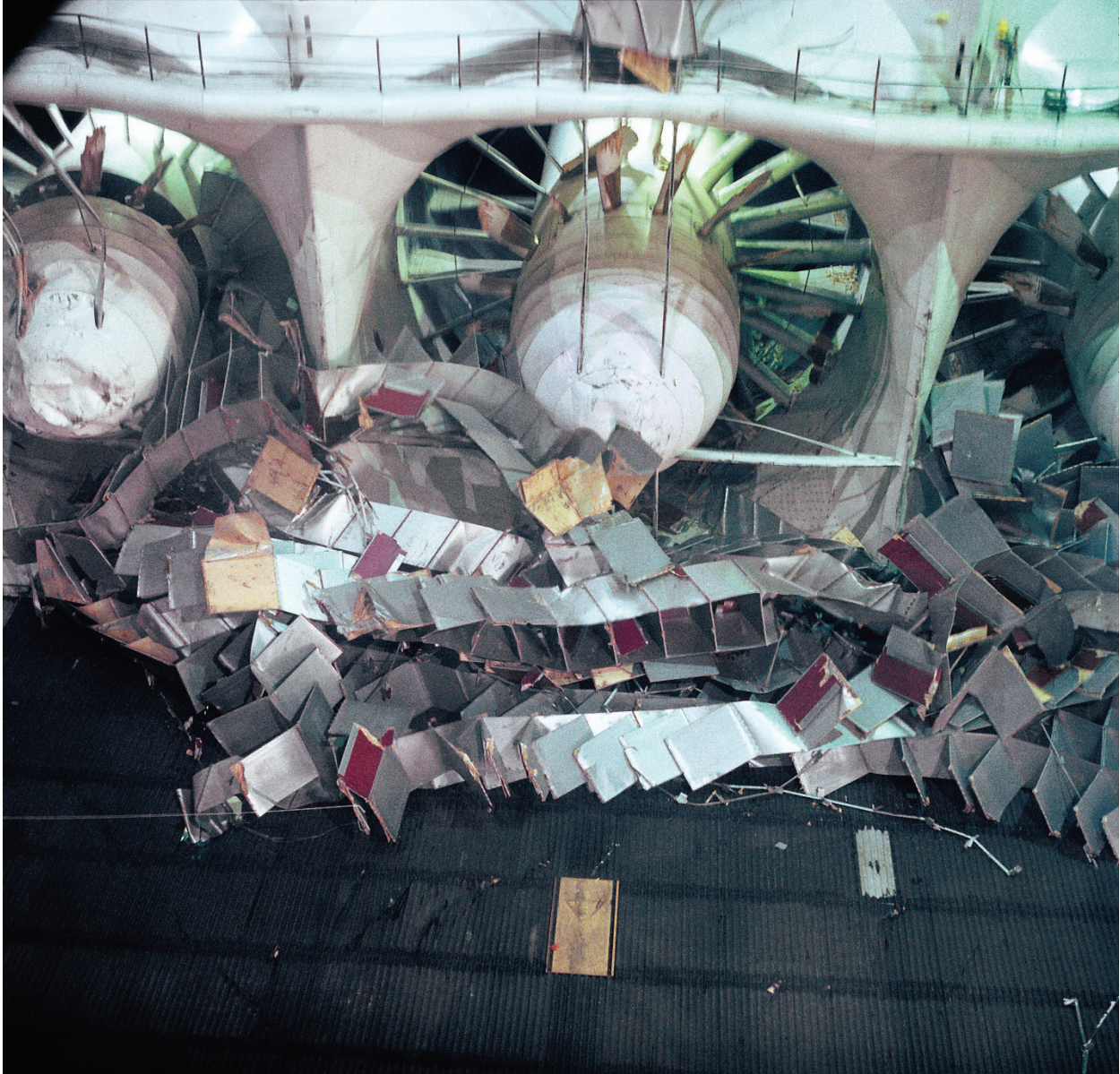
Figure 53. Results of the 1982 accident showing collapsed vane set five in front of the drive. (NASA AC82-0875-183)
