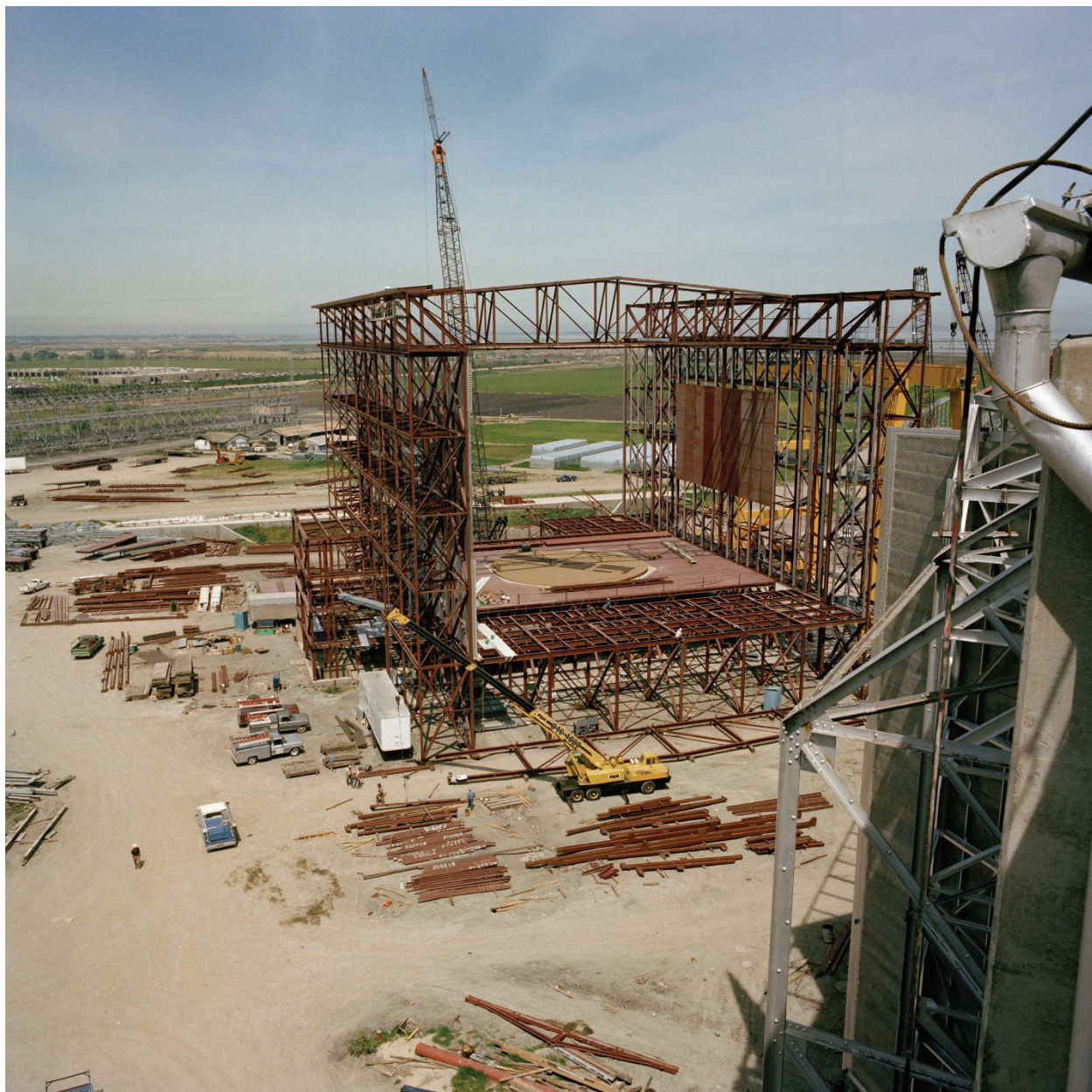
Figure 39. Beginning of the 80- by 120-foot test-section test leg framing. (NASA AC81-8017-25)
