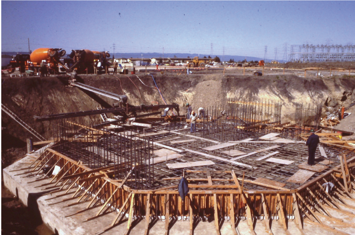
Figure 32. Beginning of concrete forms for construction of the 80- by 120-foot test-section model support and balance. ( Author's collection, KM31 )
