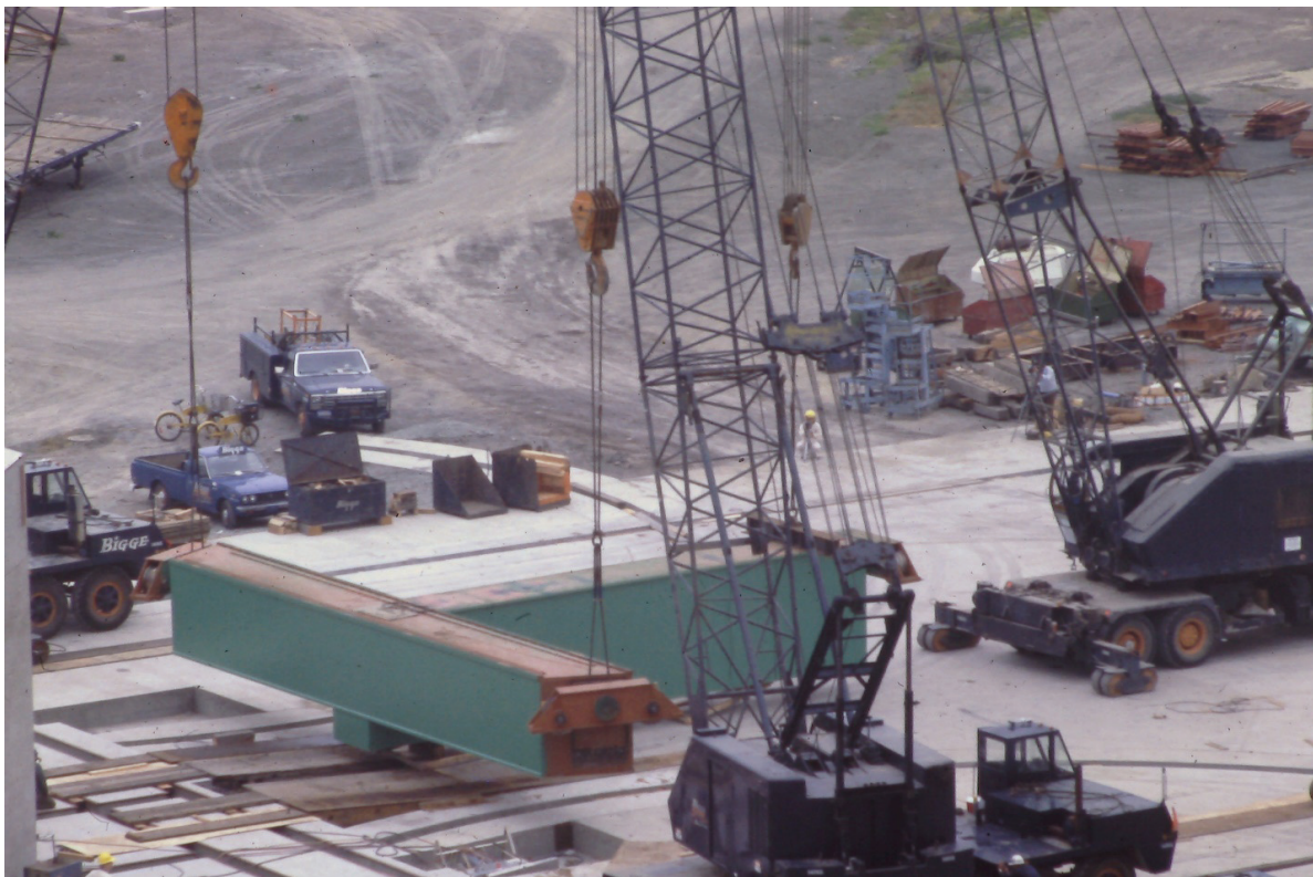
Figure 35. Lifting the model support T-frame. (Author's collection, KM39)
